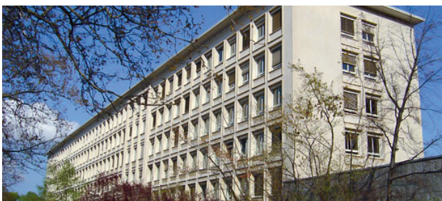
Figure 1 IEC building based in Geneva Switzerland
